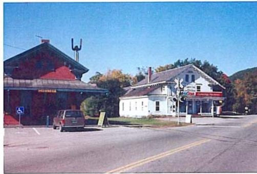
Bicycle and pedestrian facilities at bus or train stations enhance multi-modal opportunities (Chester Depot)
