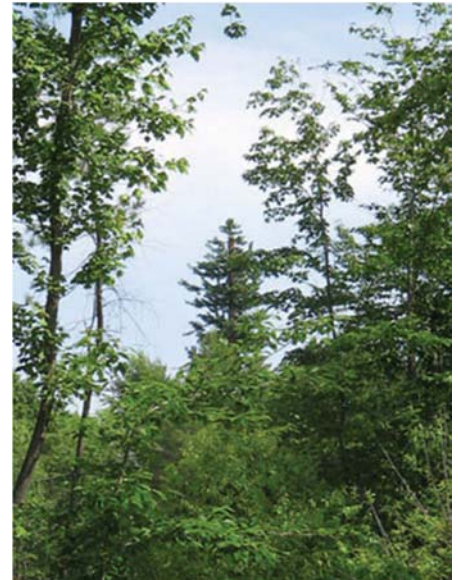
Figure 4.16.1: These photographs illustrate acceptable forms of stealth design. Note that the "monopine" towers in these two photos blend in with the surrounding trees and do not stick up above the tree line.
